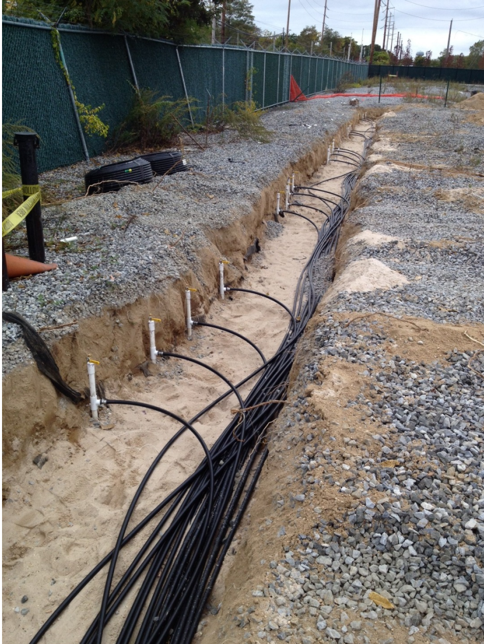
Excavated trench at OU-1 North
