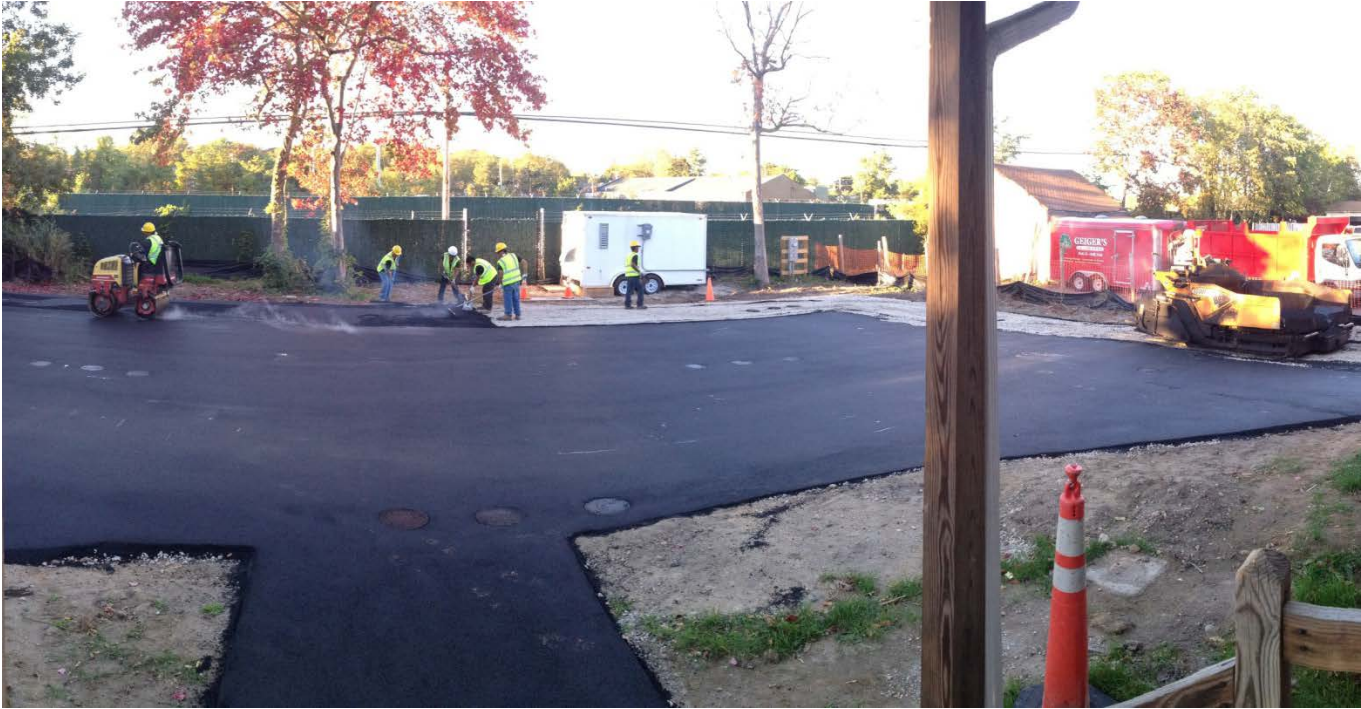
Paving at 87 Community Road
