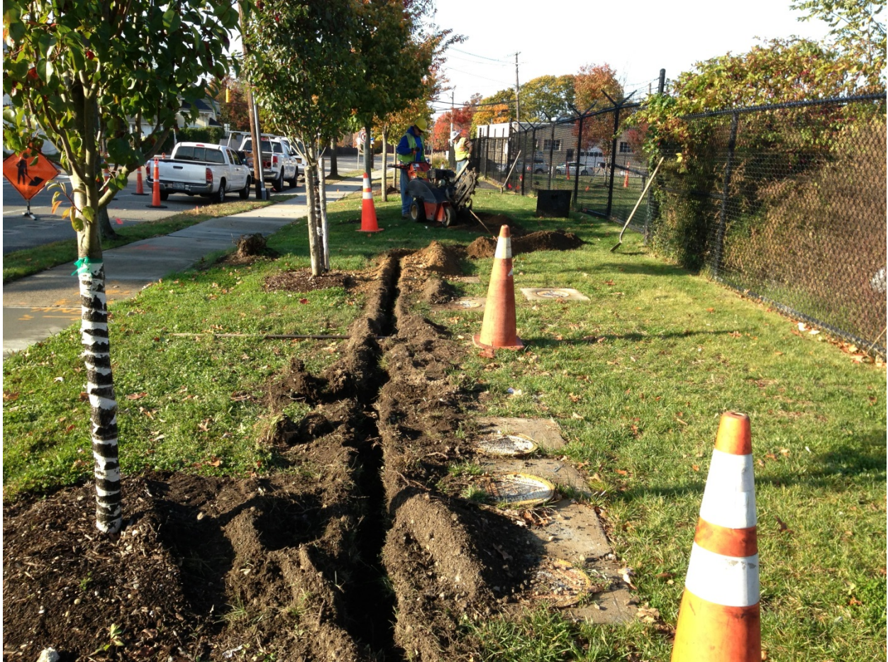
Trenching along Union Boulevard
