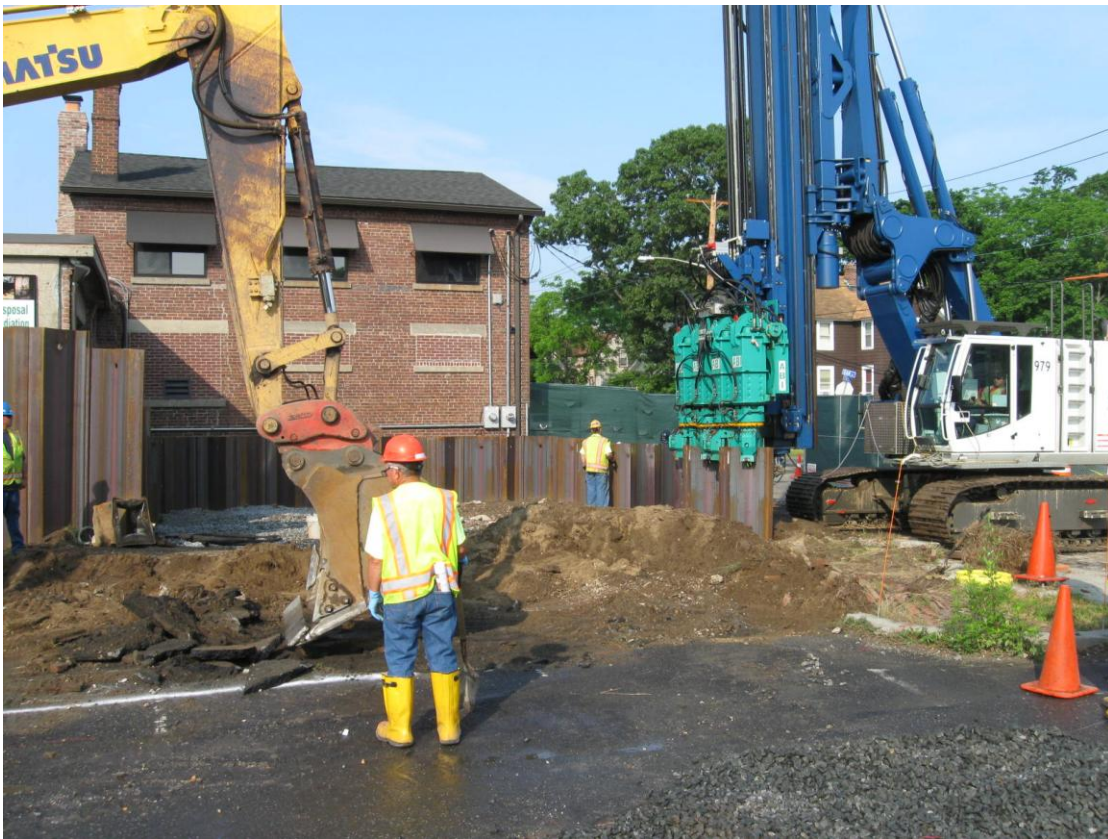
Driving sheeting and removing pavement in Phase 2
