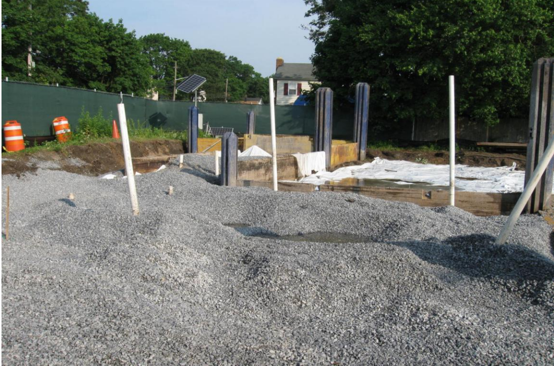
Phase 1 excavation shoring and backfill
