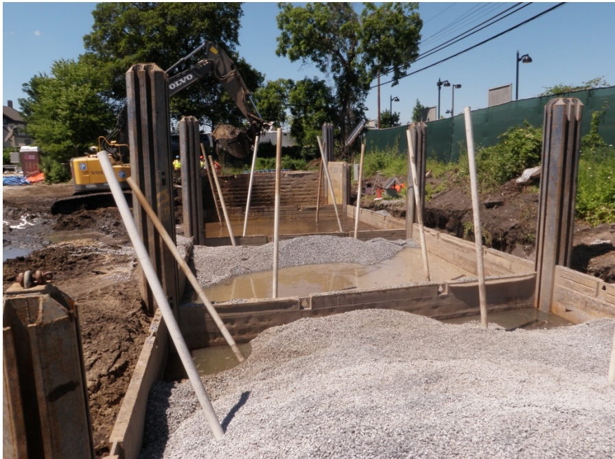
Slide rail excavation with survey poles in Phase 3
