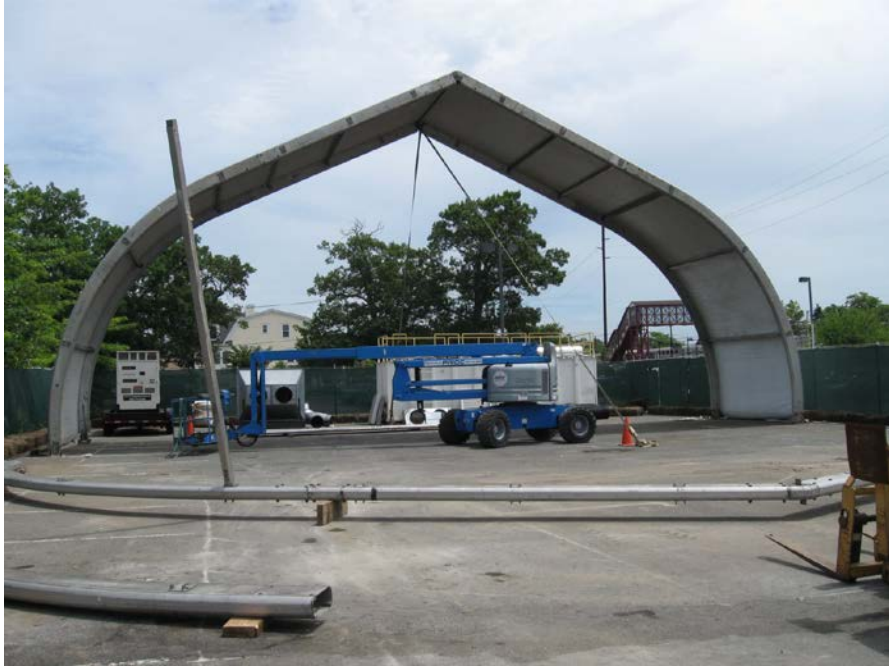
Impacted soil storage tent dismantling in Phase 2B
