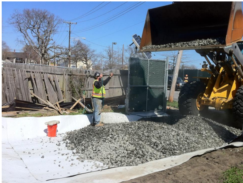
Constructing the Anti-Tracking/Decontamination Pad
