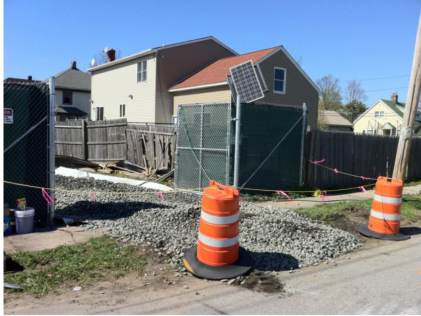
Finished Anti-Tracking/Decontamination Pad
