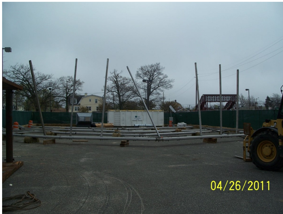
TFS construction underway
