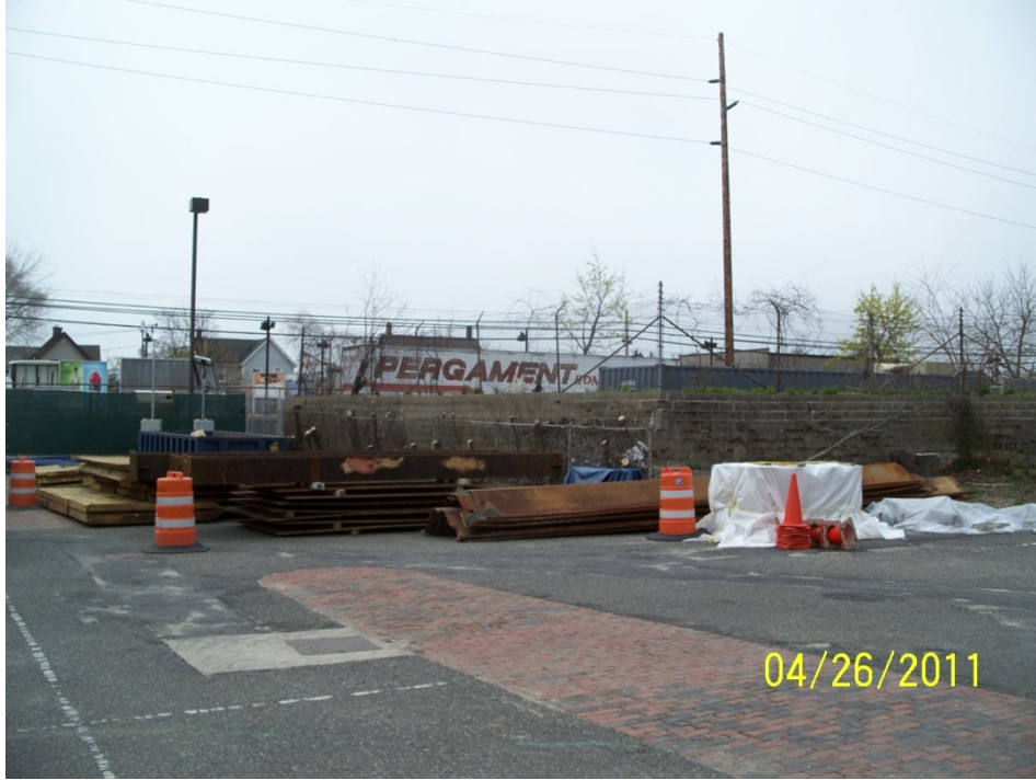
Sheet pile and shoring staged and ready for installation
