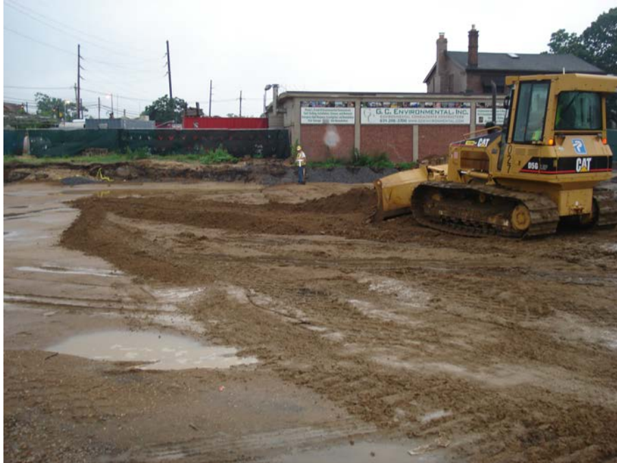
Phase 2 backfill and compaction over stone and fabric
