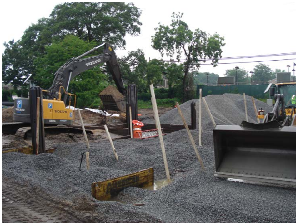
Phase 3 excavation in slide rail boxes with survey poles
