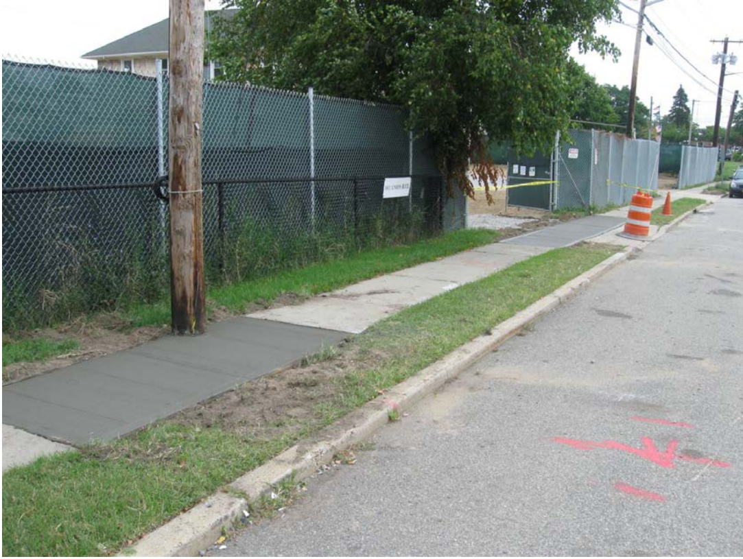
Union Street Sidewalk Restoration
