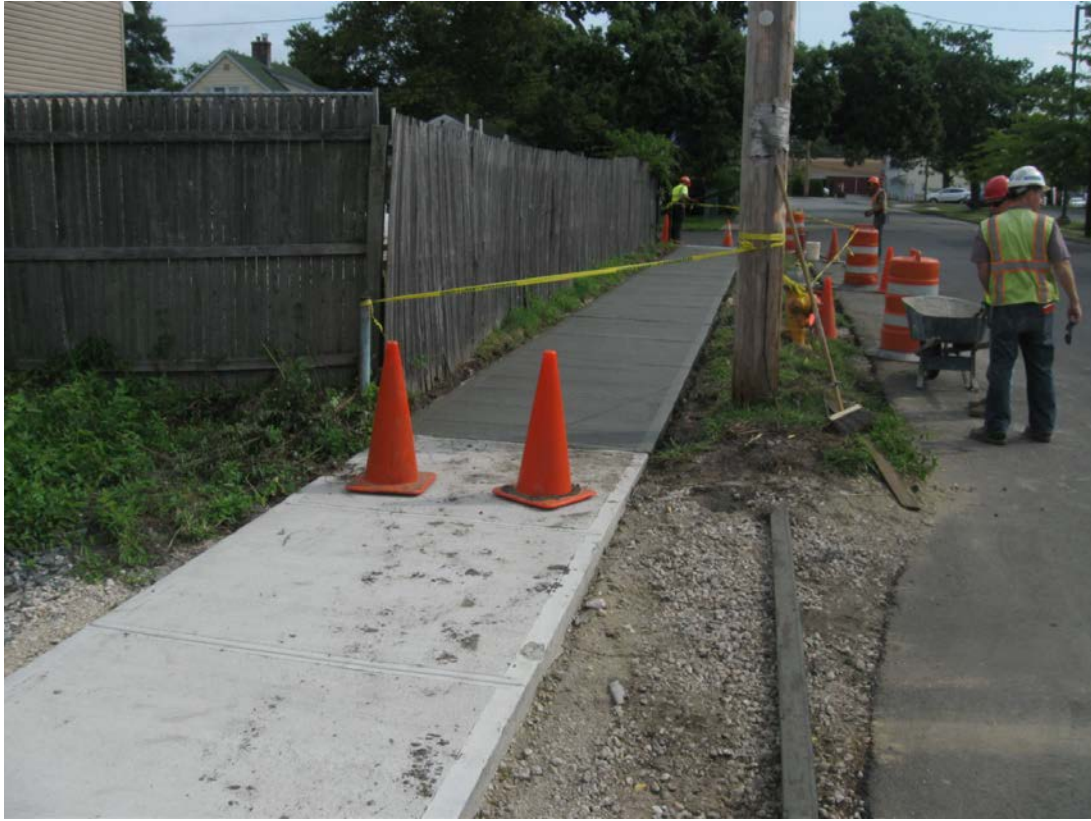
Oak Street Sidewalk Restoration.
