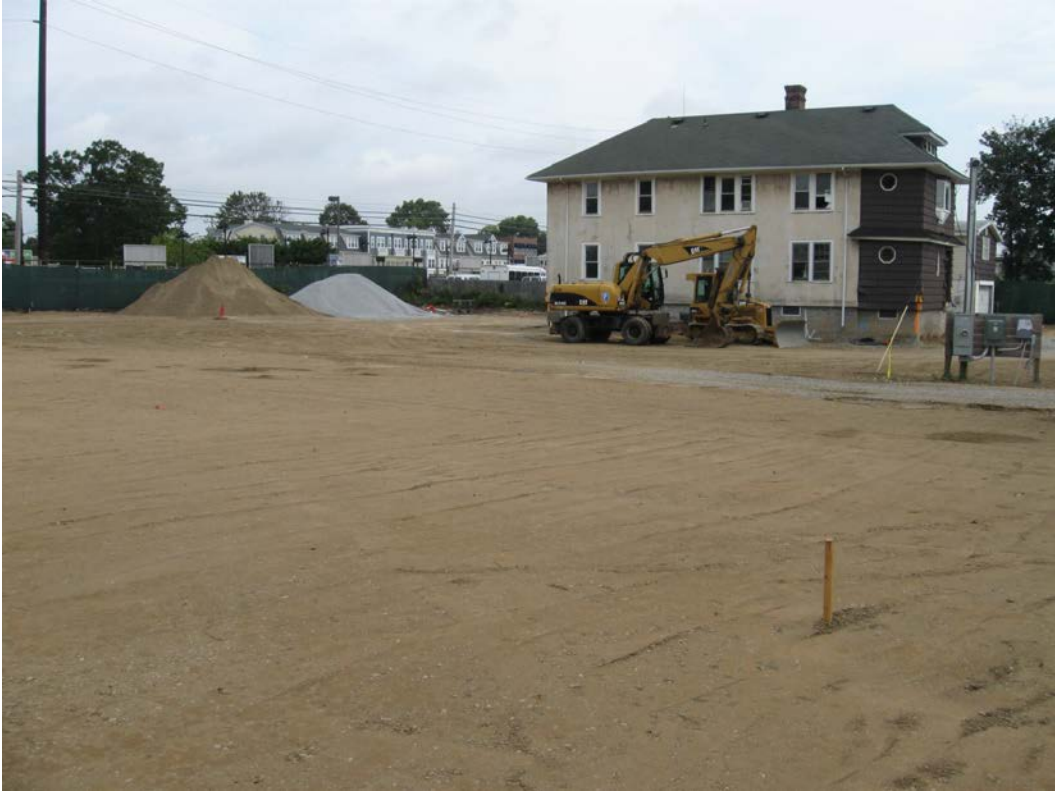
Phase 3 Backfill Complete
