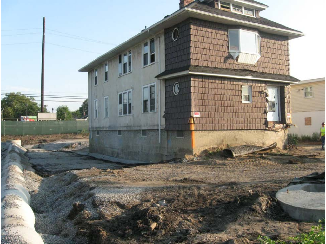
Phase 3 Shallow Excavation
