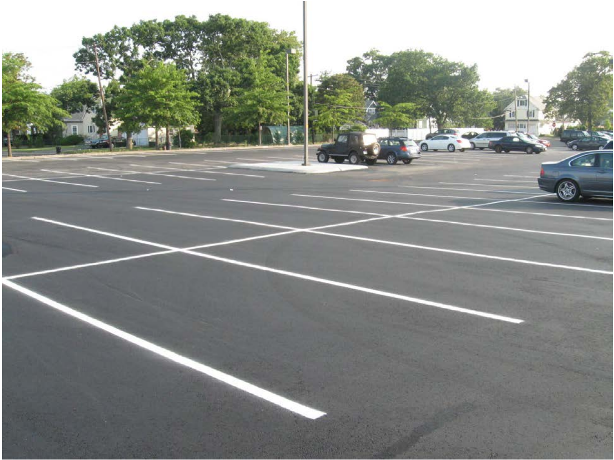
Phase 2 Restored Parking Lot
