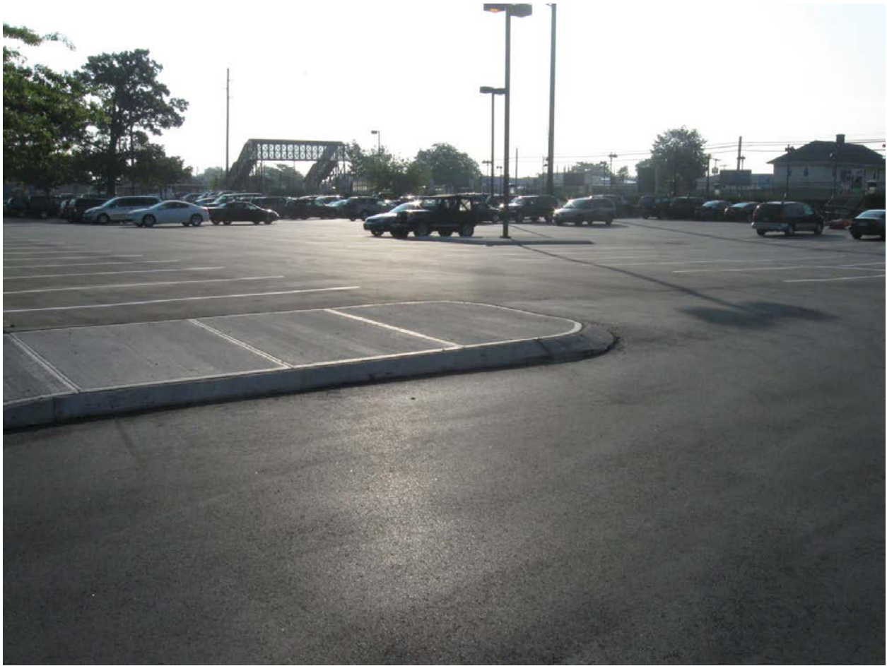
Phase 2 Restored Parking Lot
